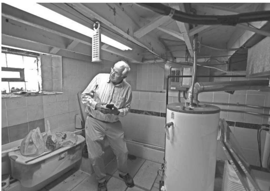
Andrew Helgeson, home inspector for Security Home Inspection Corp., prepares to check the electrical at a home in Germantown on Wednesday. Many problems in a house are invisible to the naked eye. ANGELA PETERSON / MILWAUKEE JOURNAL SENTINEL
